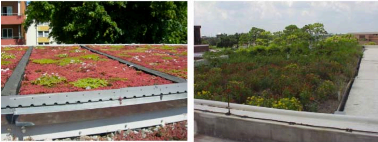
Figure 1. Left: Extensive green roof in Sweden (Berndtsson et al, 2009). Right: Intensive green roof in Florida (Sonne, 2006).
