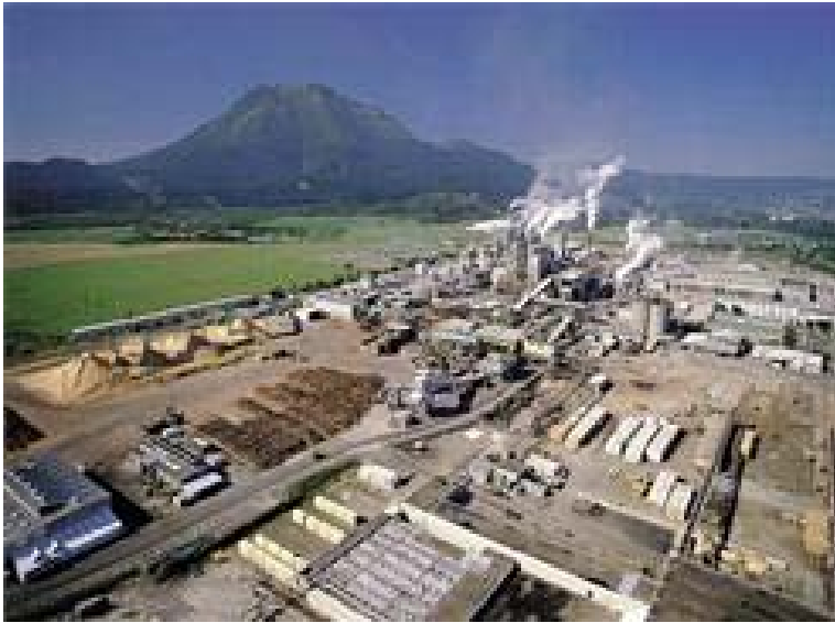
Figure 3: The production facility of the Tasman Pulp and Paper Mill in Kawerau, Bay of Plenty ( www.norskeskog.com ).
