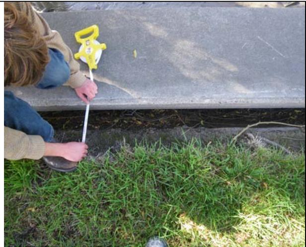
*Lateral Spreading Caused the Cut to Move Inwards and Away from the land.*
