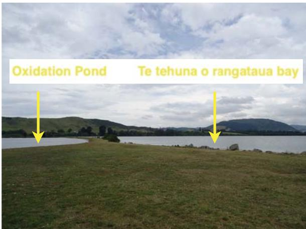
Figure 3 is a photo showing the close proximity of the pond and the harbour—approximately 5 meters at the narrowest width. During storm events washovers can instantly pollute the harbour water through leakage. Figure 4 and 5, respectively, show sewage material trapped in riparian vegetation and sewage material floating in the harbour.
